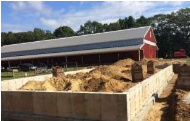
And VOILA!! By Wednesday after Labor Day weekend, the footings and foundation were done!
