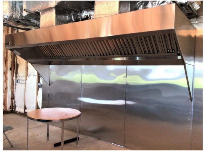
The duct work will be covered eventually.
