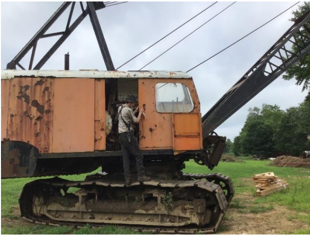
The new "crane guy", our Vice President Connor Bishop, normally found in the Engine Building. The crane was used to lift the trusses.
