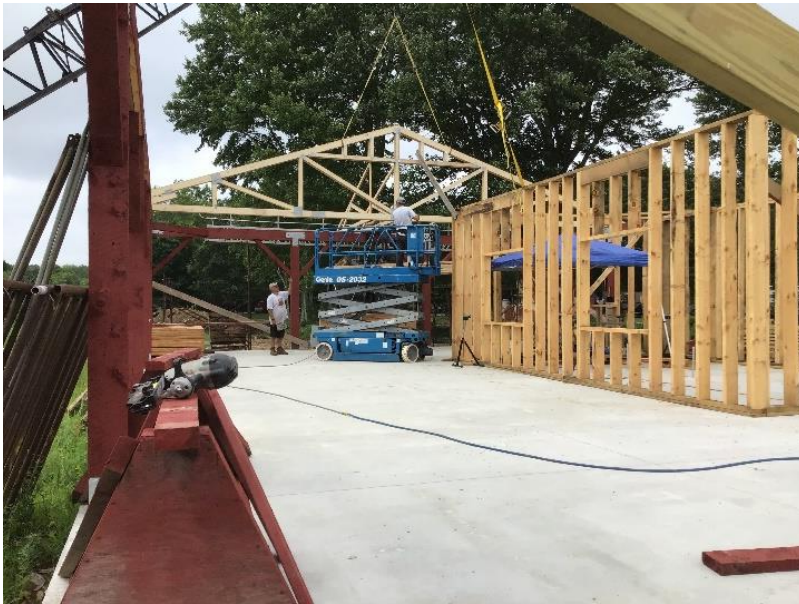
First roof truss.
